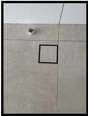
Outlet/floor trap
